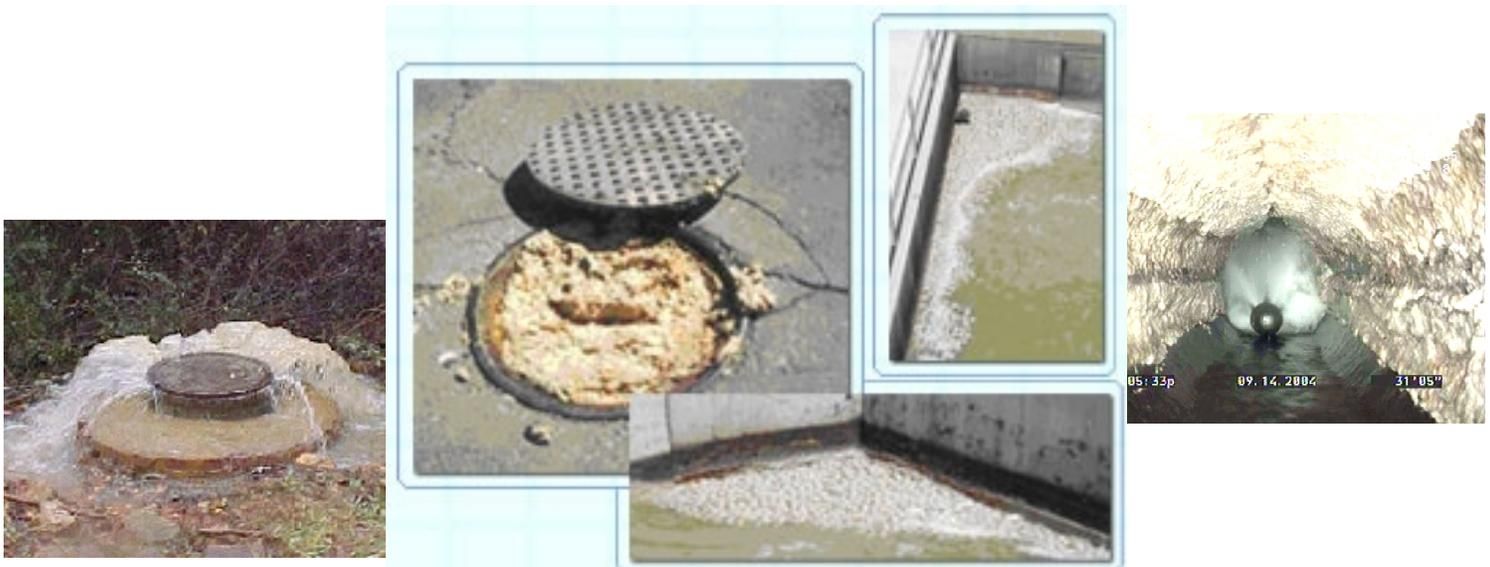
Figure: The effects of FOG accumulation in the sanitary sewer system.
